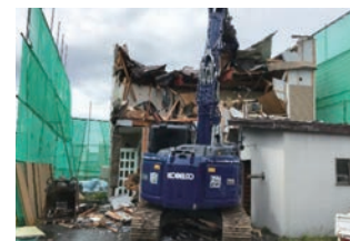
Demolition of a residential house
