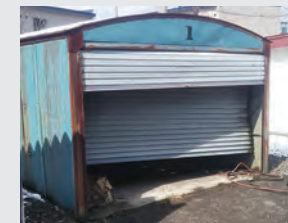
Before garage removal
