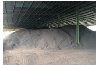
Mine Biomass Synergies PKS Stockyard
