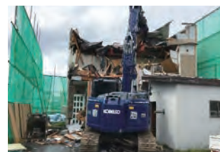
Demolition of a residential house
