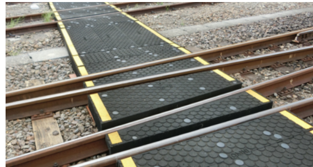
Omni-rubber panel construction of colored panels for pedestrians
