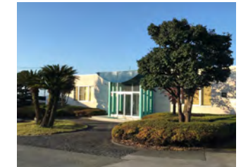
④ Toyo Rubber Chip Co., Ltd. Head office plant
