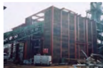
Installation of large shredder
