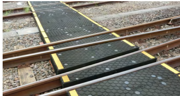
Omni-rubber panel construction of colored panels for pedestrians
