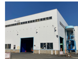
⑦ VOLTA Inc. Head office plant
