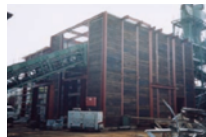
Installation of large shredder
